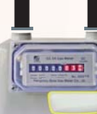
Energy monitoring Gas
